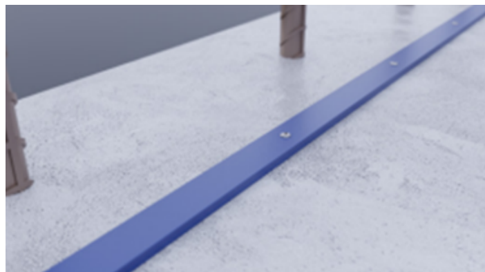
MECHANICALLY ANCHORED BEAD
