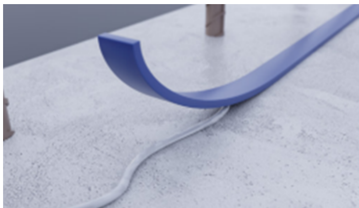
ADHESION THE BEAD WITH PUMALASTIC MS
